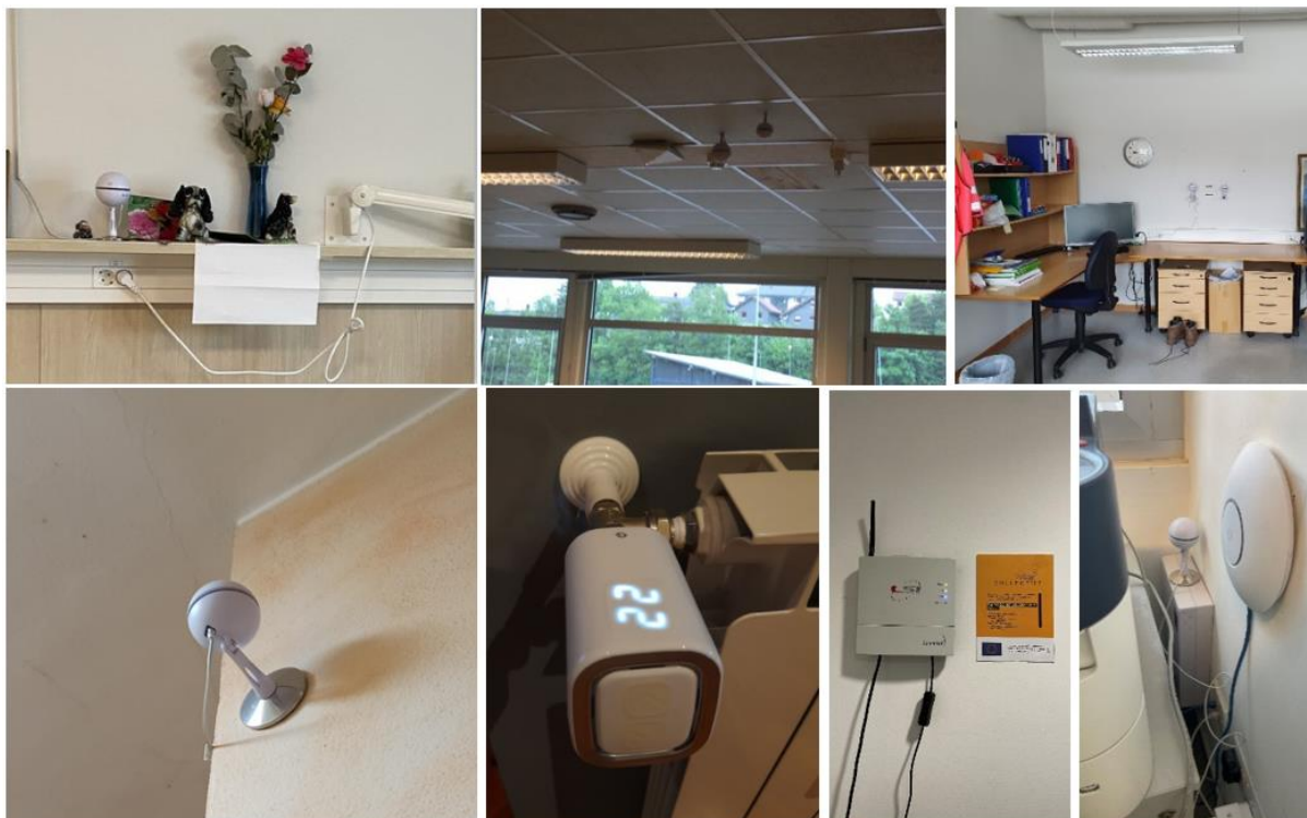
Figure 9 Photographs of the installation of Sphensors, BRiG, Smart Plugs and Valves in the pilot buildings
